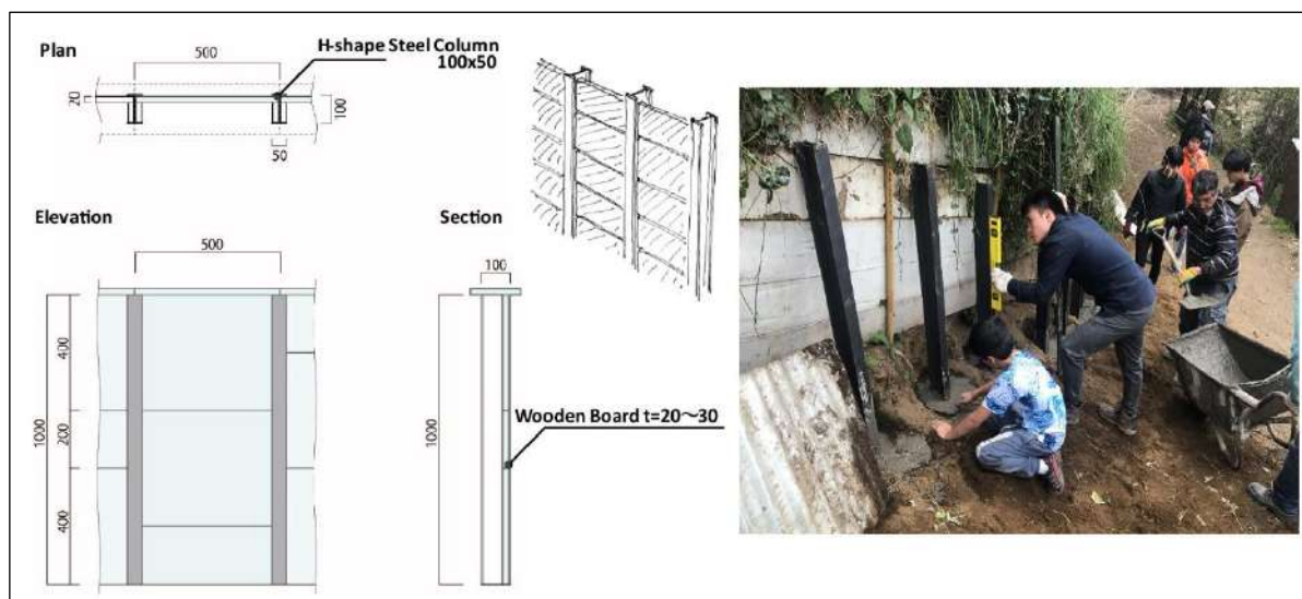
Figure 10. Piled Soil Wall Construction System
